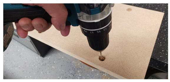
**Step 7:** Flip over the Wasteboard strip so the counter bore holes are facing down. With the wasteboard strip flipped over, drill open the 1/16" holes you drilled in step 6 using a 1/4" Drill Bit.
